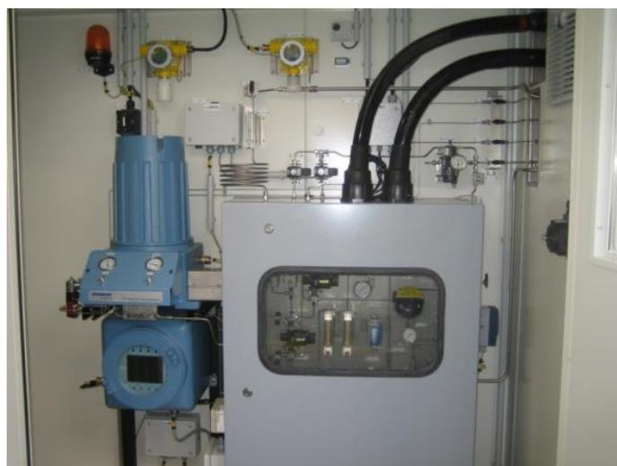
Figure 63. Gas chromatograph used at the Bioliq plant by KIT [159].
