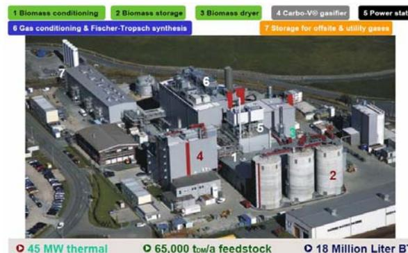
Figure 5: Choren  $\beta$ -plant Freiberg - BtL production in semi industrial scale [33]
