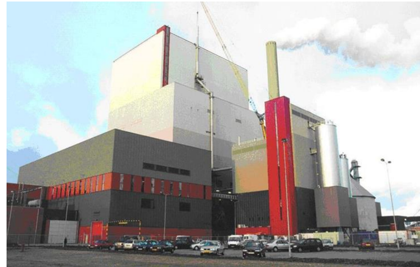
The Amer-9 coal-fired power station with the waste wood
