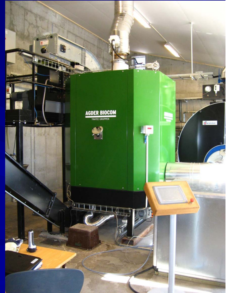
Wood Technology Research Centre
