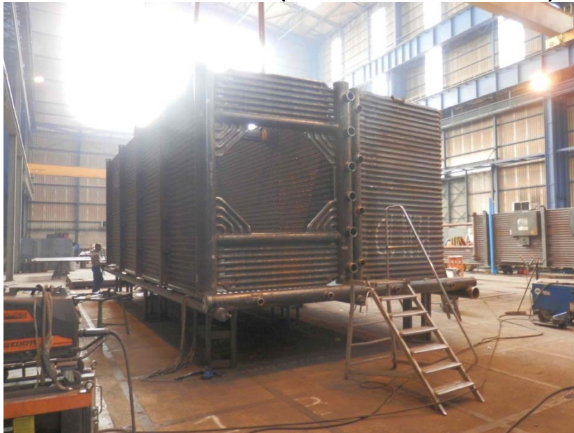
Waste heat boiler (under construction)
