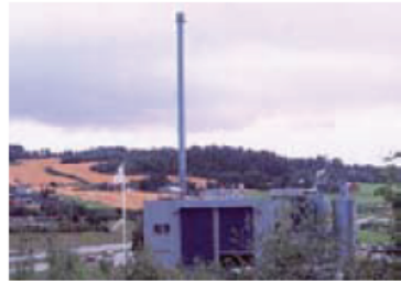
Ranheim Plant Location: Norway Commissioned: 1997 Fuel capacity: 10,000 tonnes/year Energy production: 25 GWh (thermal)/year
