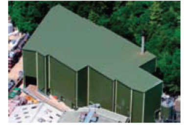
Isle of Wight Plant Location: United Kingdom Commissioned: January 2009 Fuel capacity: 30,000 tonnes/year Energy production: (electrical) 1.8MW
