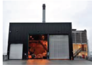
Forus Plant Location: Norway Commissioned: 2002 Fuel capacity: 39,000 tonnes/year Energy production: CHP 105 GWh (thermal)/year
