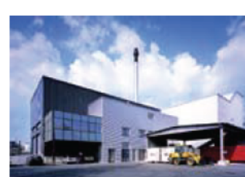
Minden Plant Location: Germany Commissioned: 2001 Fuel capacity: 39,000 tonnes/year Energy production: 105 GWh (thermal)/year
