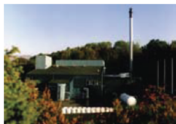
Averøy Plant Location: Norway Commissioned: 2000 Fuel capacity: 30,000 tonnes/year Energy production: CHP 69 GWh (thermal)/year
