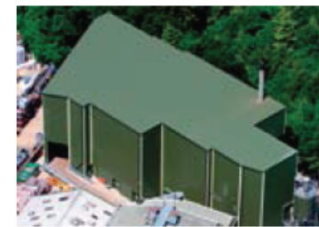
Isle of Wight Plant Location: United Kingdom Commissioned: January 2009 Fuel capacity: 30,000 tonnes/year Energy production: (electrical) 1.8MW
