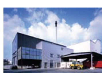
Minden Plant Location: Germany Commissioned: 2001 Fuel capacity: 39,000 tonnes/year Energy production: 105 GWh (thermal)/year
