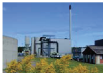
Sarpsborg1 Plant Location: Norway Commissioned: 2002 Fuel capacity: 78,000 tonnes/year Energy production: 210 GWh (thermal)/year
