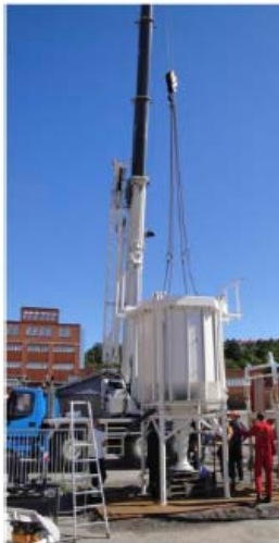
Construction of the plant
