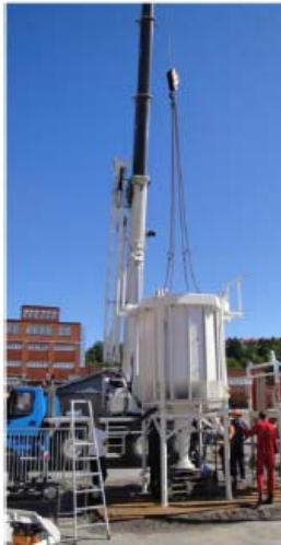
Construction of the plant
