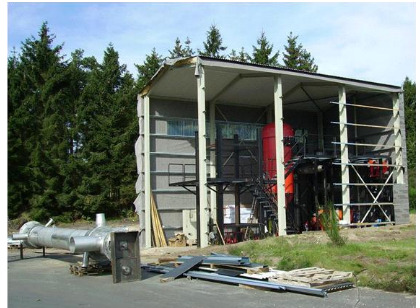
Installation of 200kW gassifier in Hadsund (DK)
