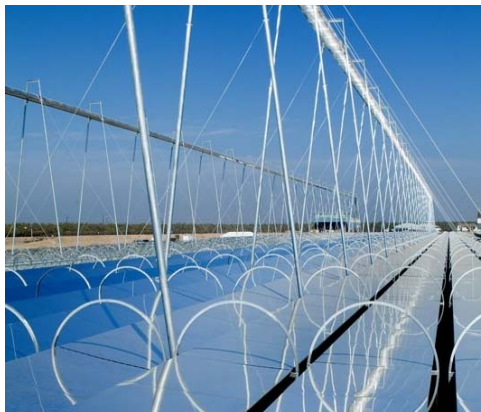
Linear Fresnel Reflector (C ≈ 50, T ≈ 300 – 500 °C)
