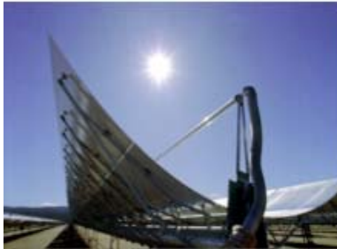
Parabolic Trough (C ≈ 80, T ≈ 400 °C)
