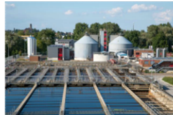
Waste water treatment plant
