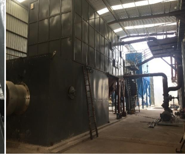
Organic heat carrier boiler
