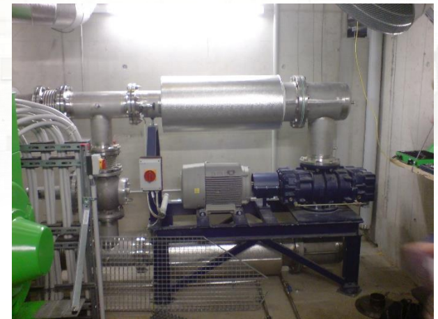
rotary piston compressor
