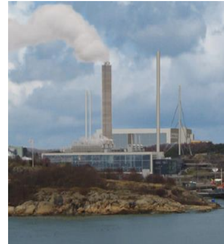
GoBiGas Phase 2 80-100 MW bio-methane Commercial Plant
