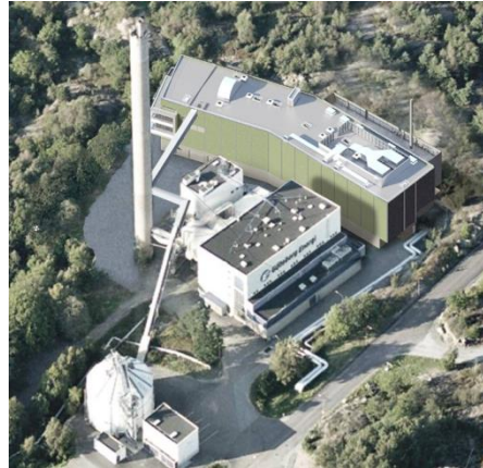
GoBiGas Phase 1 20 MW bio-methane Demonstration Plant
