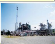
LanzaTech's Freedom Pines biorefinery (USA) for ethanol production from syngas fermentation.
