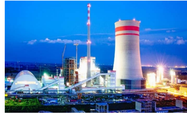
350MW SC CFB boilers in Guojin Power Plant
