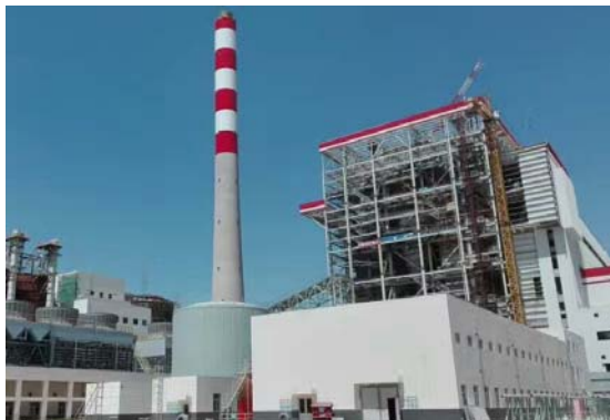
350MW SC CFB boilers in Datuhe Power Plant
