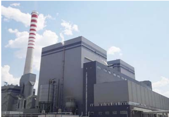
350MW SC CFB boilers in Hequ Power Plant
