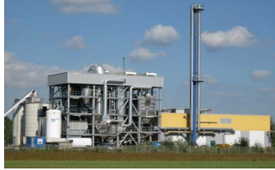
8.5 MW commercial plant Oberwart
