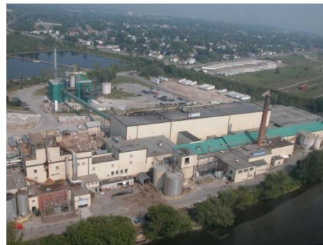
TRI BL gasifier (top left) at Norampac's Trenton, Ontario plant
