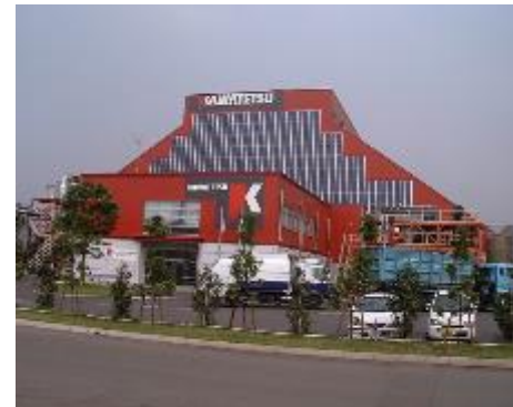
Japan Recycle Center (Chiba) 1 x JMS 620 Installed: Oct/2001 Electrical Output: 1.9 MW
