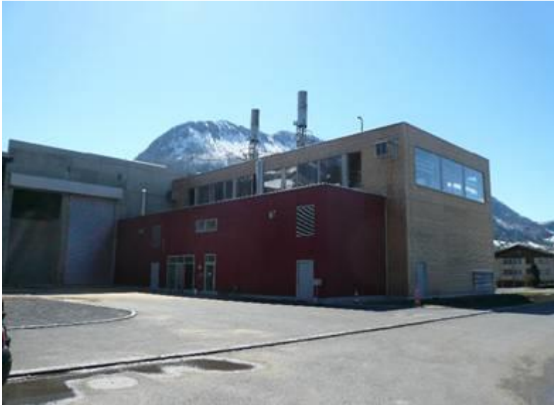
Biomass power plant Nidwalden/CH
