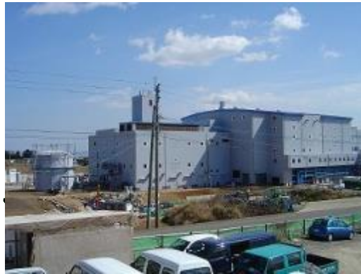
Chuo Kooiki Env. Center (Yoshino) 2 x JMS 612 Installed: May/2005 Electrical Output: 1.8 MW
