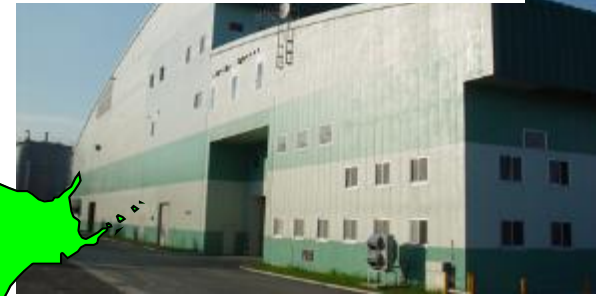
AX Green (Mutsu) 2 x JMS 616 Installed: Feb/2003 Electrical Output: 2.4 MW
