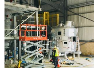
Demonstration plant furnace assembled for alignment.
