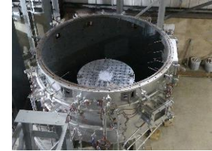
Demonstration plant furnace base - awaiting refractory lining.
