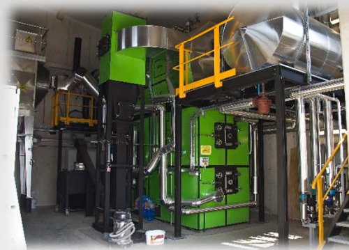
CHP by steam process up to several MWel power
