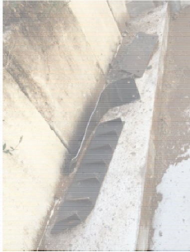
Broken backstays due to bad concrete
