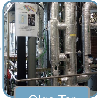
Olga Tar Removal
