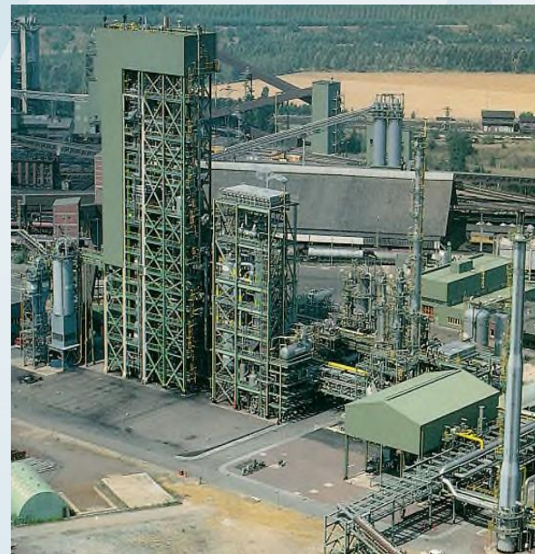
HTW Demonstration Plant Berrenrath
