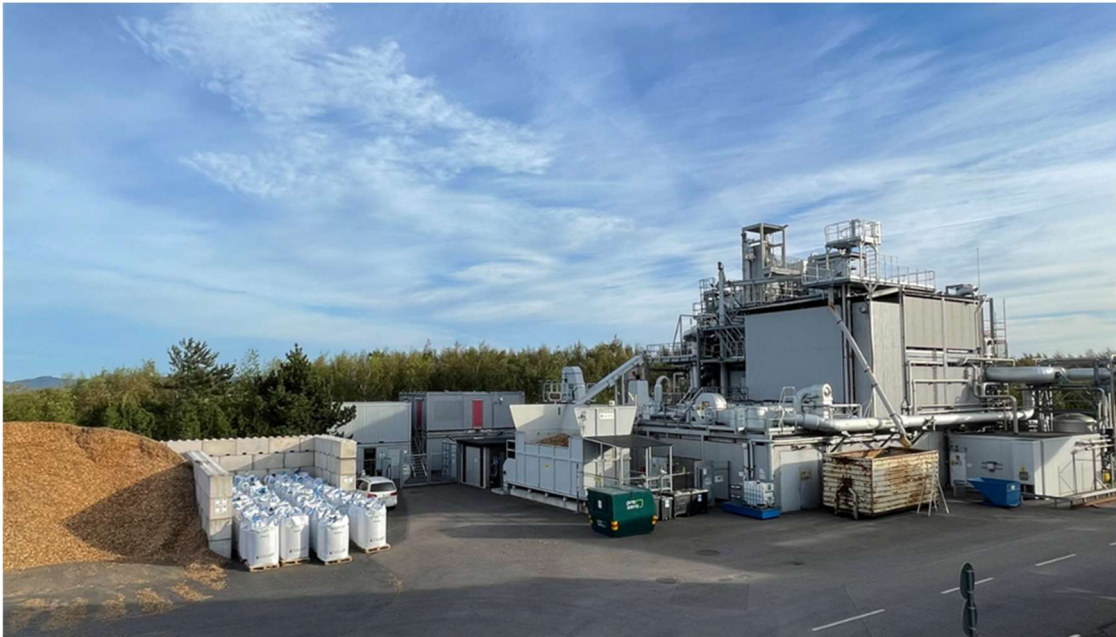
Figure 5. The WoodRoll® plant in Höganäs, Sweden (Photo from Cortus, 2024)
