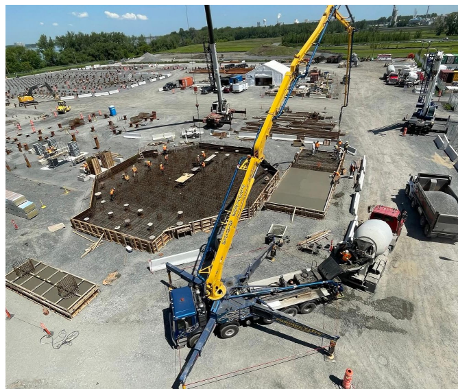
Figure 14: Construction of Enerkem facility in Varennes
