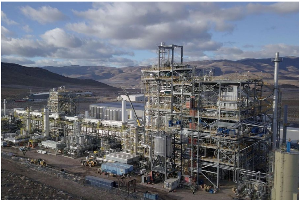
Figure 15: Sierra Biofuels - plant construction activities (May 2022)
